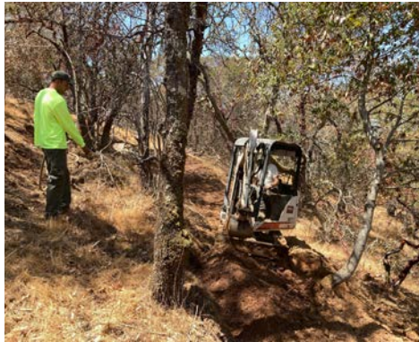
MCP crew members work with mini excavator and water line to construct the Blue Oak Trail bench cut at Rush Creek Preserve.
