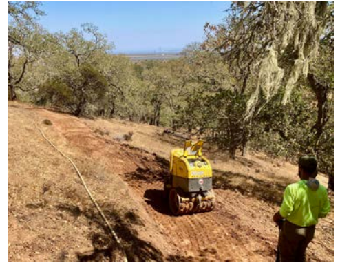
MCP crew member walks behind and remotely operates a vibratory compactor to harden the Blue Oak Trail tread.
