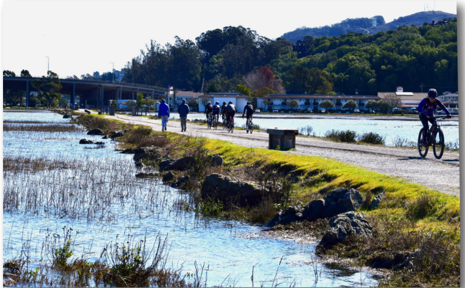
Mill Valley-Sausalito Multiuse Path will be realigned to address tidal flooding due to sea level rise.
