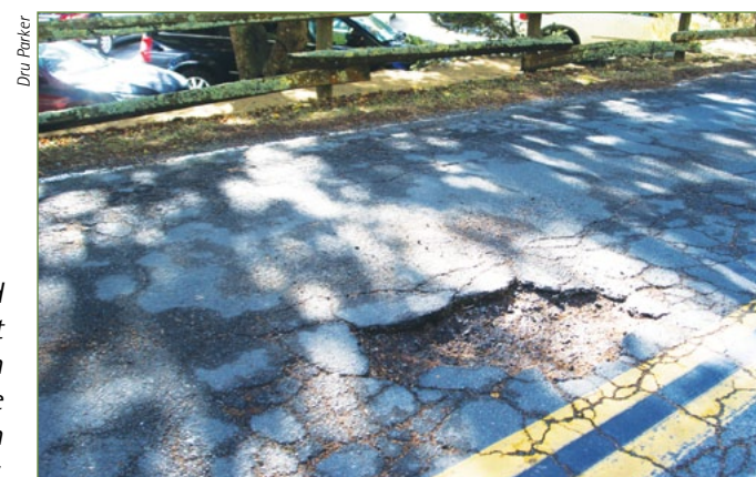
The Muir Woods Road Rehabilitation Project will repair broken asphalt and replace old culverts through Franks Valley.
