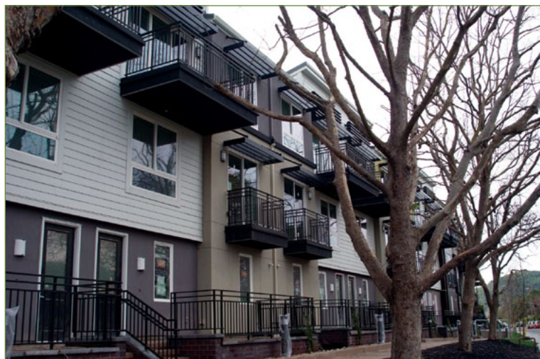
Units at Tam Ridge Residences, located at the site of the former WinCup factory in Corte Madera, will soon be ready for occupancy.
