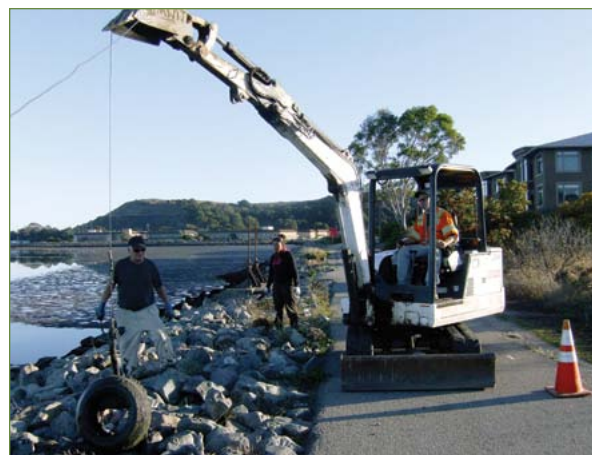
Above: Workers use a winch to remove the tires from the mud. Below: Conservation Corps North Bay workers scrape thick Bay mud from a tire.
